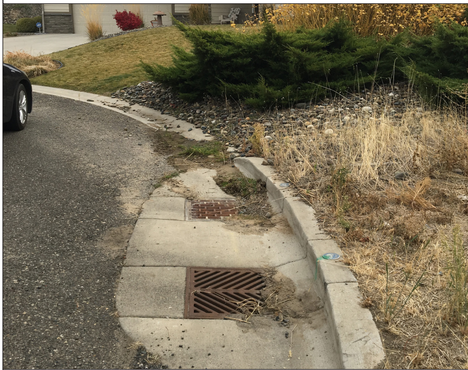
Problem Area #3 - Sediment plugging at the end of Deer Pointe Drive.
