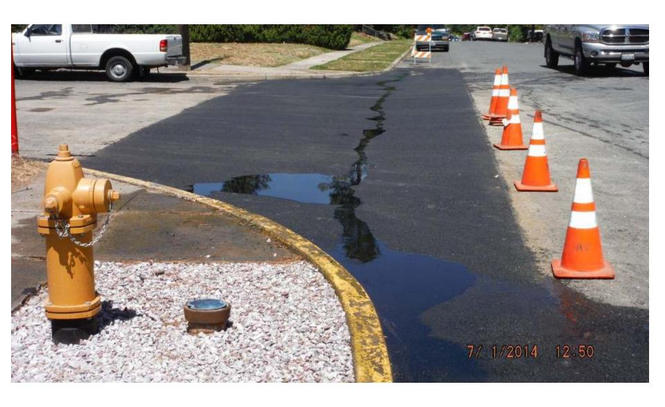
The 2 Catch Basins that spill into this drainage had been creating tremendous undercuts into the hillside where they spilled out approximately 15ft behind the curb lines.
