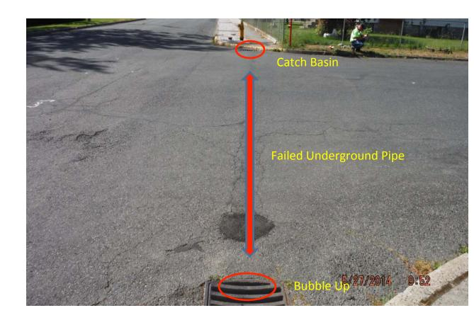
It was decided that both structures and the failed underground pipe would be removed and replaced with a cross swale similar to the one we had just done on Deer Pointe.
