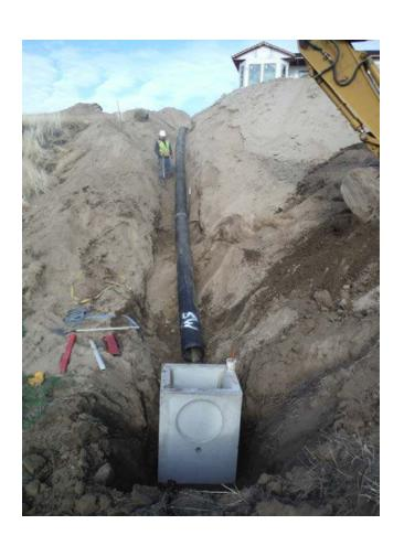
Outfall needed to be extended into the bottom of the draw and piped into a new bubble up.
