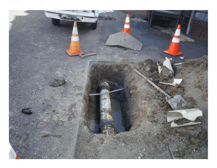
It was then backfilled, compacted and patched back with asphalt.
