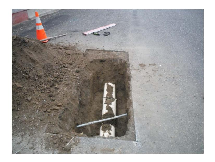
The pipe was repaired and the conduit shifted over the top of the stormwater pipe.
