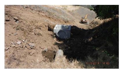
After completion of the job, the area was hydro-seeded to negate any runoff caused by disturbance of the soil.
