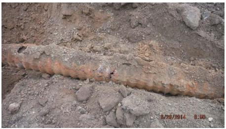
After setting grade on the drain line, the area was backfilled and compacted in preparation for asphalt.
