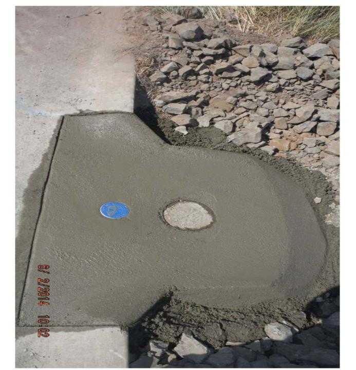
A cross drain across the roadway was installed improperly and was causing a traffic hazard.
