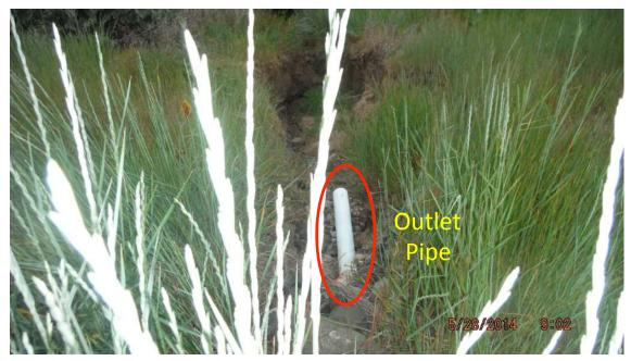
Over the course of time and constant water flow, the pipe outlet eroded away a considerable sized hole.
