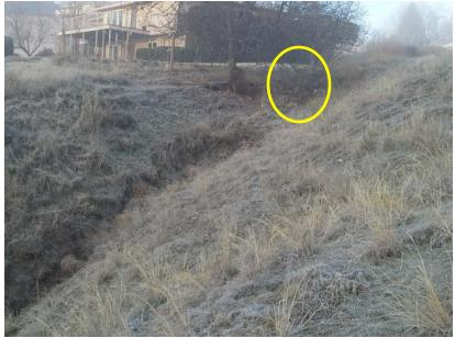
It was decided that the best solution to this problem would be to pipe both Catch Basins into a Bubble Up structure at the bottom of the natural drainage.
