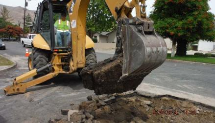
Next the existing structures were removed, along with the failed underground piping.
