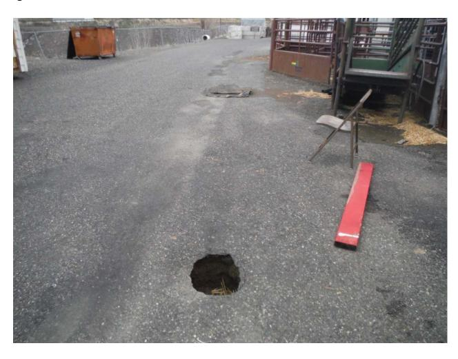
It was determined that when the electrical conduit was run to another building behind the problem area, it was bored through the existing stormwater pipe.
