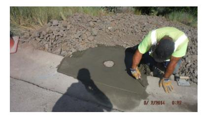
A riser for a PUD water valve was dead center in the low area where the spillway needed to be.
