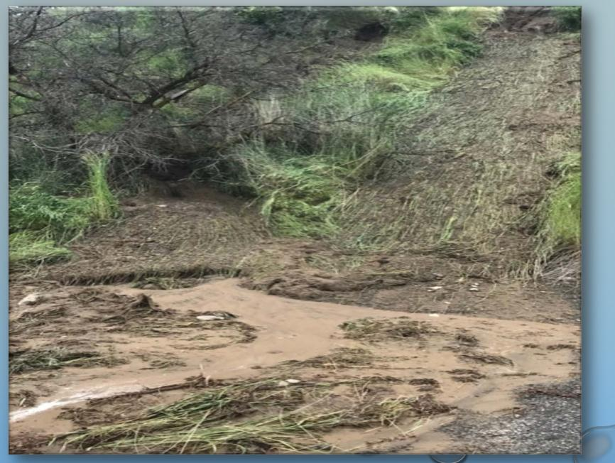
DRAIN-GRATE BECAME CLOGGED WITH DEBRIS AND WATER WAS NOT ABLE TO FLOW INTO STORM SYSTEM.
