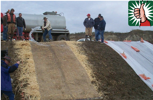
An example of slope stabilization of exposed dirt using straw and plastic.
